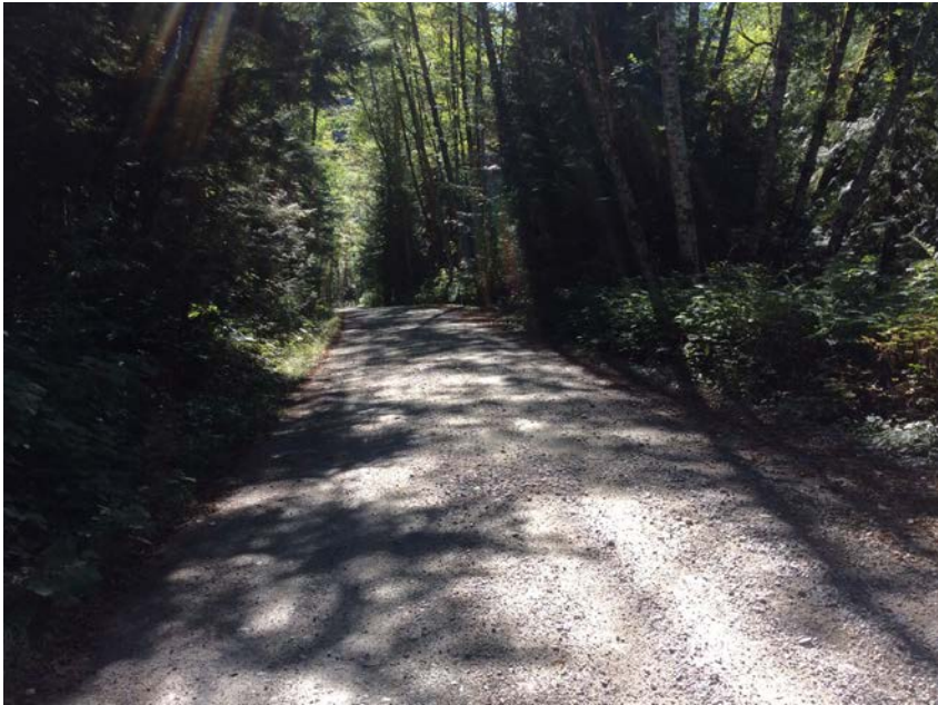
Left approach viewed from bridge
