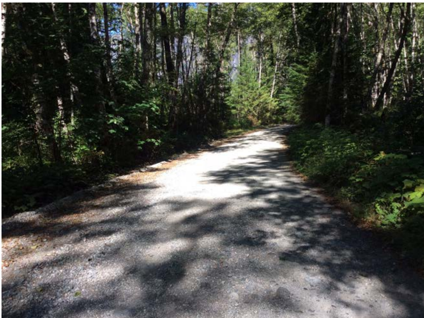
Right approach viewed from bridge
